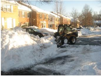
One final observation: Fire hydrants were covered up as snow was piled on the peninsulas and other common areas. Make sure fire hydrants are always accessible to the Fire Service. Should a house catch on fire, severe damage could be done not only to that house but to adjacent dwellings if firemen have to spend extra time digging the fire hydrants out.
